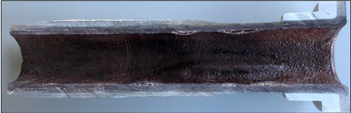
Figure L7. The online monitored pipe section showed severe material corrosion, which led to a changed signal for the lamb wave propagation.
